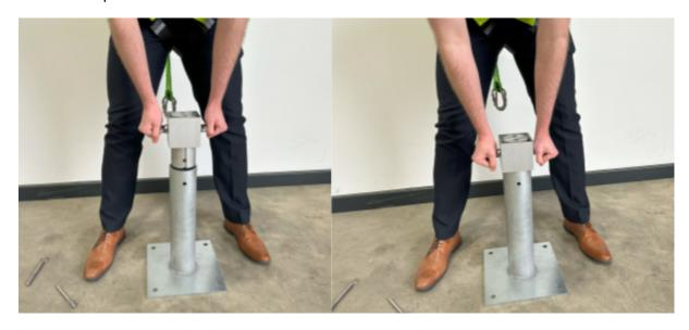
**Step 2**Securely pin in two places structural
