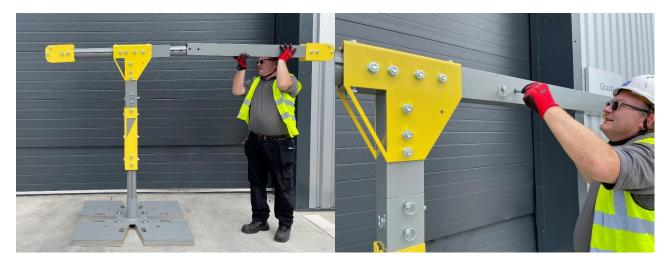
Slot component 3 onto component 2 and ensure security by inserting 2 Mx16 quick release pins in the side and 1 Mx16 quick release pin through the top. Rotate the davit back into position if required and insert an Mx12 quick release pin through the davit base and component one if using DBS-0300-0200 or DBS-0400-0300 to fix the davit arm in place and prevent rotation during use.
