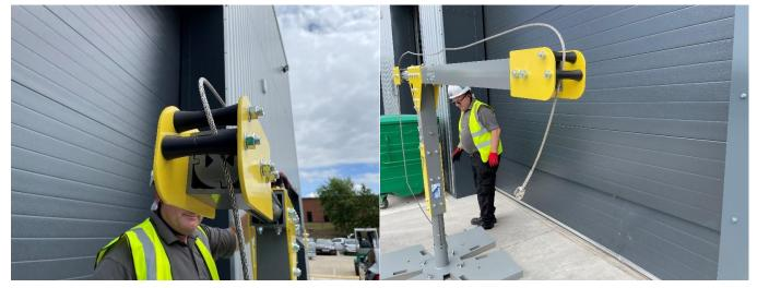
When rigging, ensure that the rope is passed between both rollers at both anchor points. The rope must pass over the davit.
