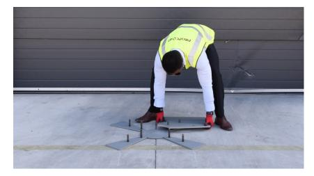
Following step 2, place one of the top counterweights on top of each wing of the assembly. They can be guided down and positioned correctly using the threaded rods.
