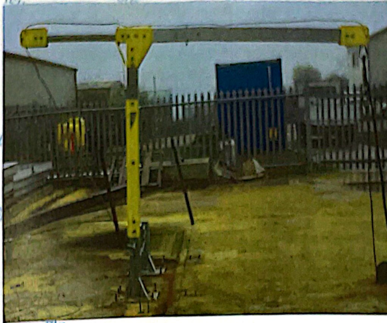
Figure 1 – Anchor described as "2500 x 2500 davit arm"
